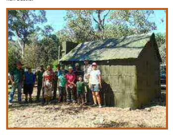
The working group replaced some old weather beaten mini corrugated iron, and a support beam, with replacement (second-hand) mini-corrugated, iron similar to what was originally on the hut, fixed up and re-mortared the fireplace inside and repainted the outside of the hut.
